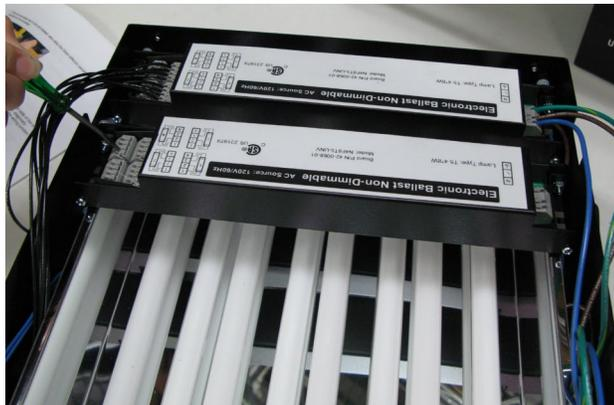
10. Working wire by wire, repeat these steps until all wires have been transferred from the old to the new ballast, taking care to match the location of the wires from the old to new ballasts. Note that there are wires which must be transferred on both sides of the ballast.
