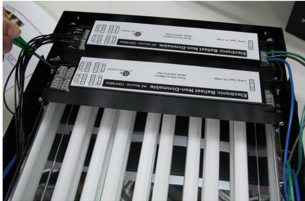
8. Grasp one of the wires inserted into the gray plastic wiring junction on either side of the old ballast. **Noting the location of the wire**, press down on the spring loaded, diagonally-hashed wire retainer with a flat head screwdriver to release the wire from the wiring junction.
